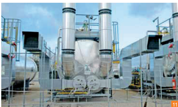
[8-9-11] Indirect Bath Heater // Client: Ansaldo // Place: Aprilia (Italy)
