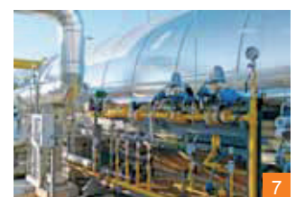
[1-7] Indirect Bath Heater // Client: Ansaldo // Place: Aprilia (Italy)
